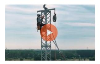
Following the fierce storm that crossed Belgium on 9 July, Elia's teams have now built five backup pylons and integrated them into the grid. This backup line was erected in record time. It will remain in service until the high-voltage line that was damaged by the storm is up and running again. The storm caused nine high-voltage pylons to fall over into fields and onto 15 homes in Leest near Mechelen.
